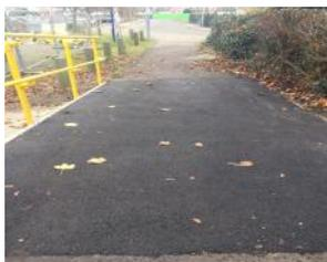
**Fig 4: The refurbished path to Platform 2. Note the lack of textured paving at the top.**
